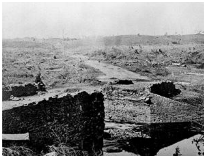
Ruins of Stone Bridge at Bull Run Creek, Manassas, Virginia, March 1862.
